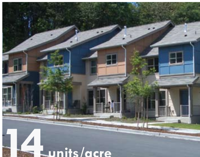
These townhouses at the Rainier Vista mixed-use development in Seattle provide eight low and moderate-income homes on 0.6 acres for a net density of 14 units per acre.
