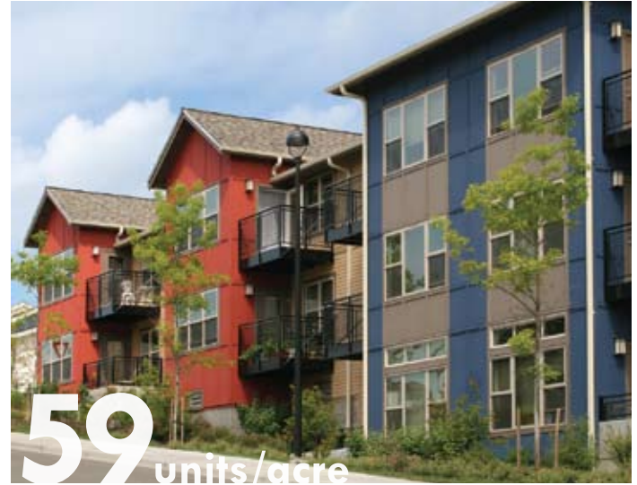
The Nia Apartments at the Greenbridge mixed-use development in White Center provides 82 low-income apartments on 1.39 acres for a net density of 59 units per acre.
