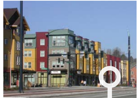
Housing Affordability: The moderately dense Rainier Vista Hope VI development in Seattle provides a range of low, moderate and market rate ownership and rental units adjacent to light rail.
